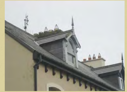
Dormer attic with timber spear finial
