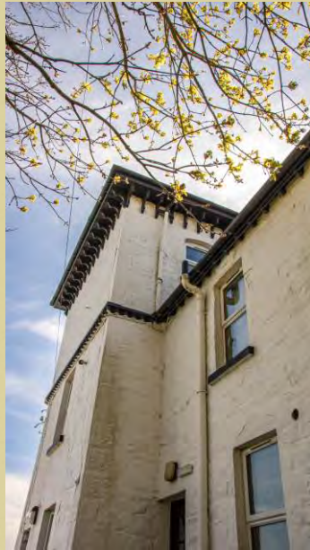
Mildly battered (sloping) three-storey tower with dogtooth string course and corbelled eaves above
