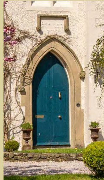
Sandstone surround with hood moulding
