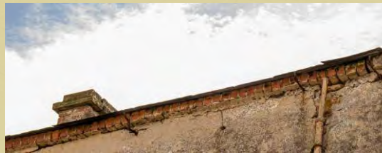
Brick eaves course
