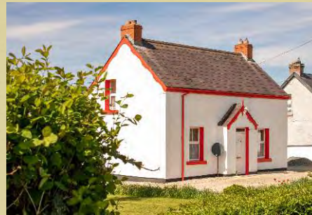
Decorative bargeboards to gable and porch
